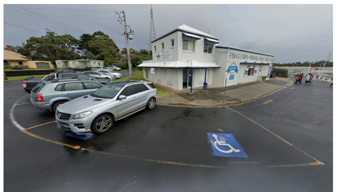
Figure 43 Kerb ramps are obstructed by vehicle in accessible parking bays
