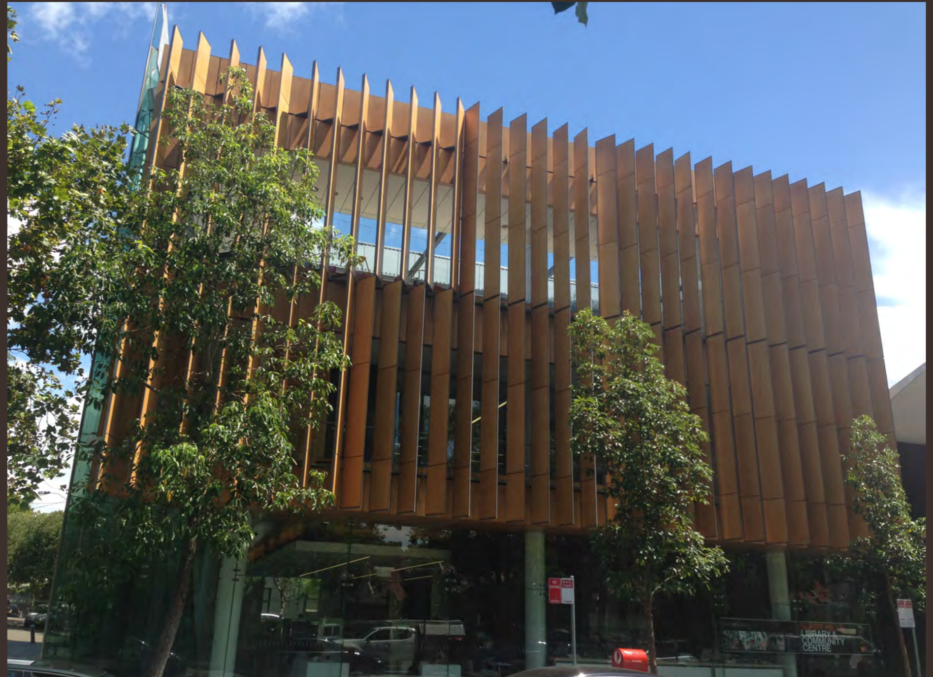
A new landmark building would attract visitation and activate the town square
