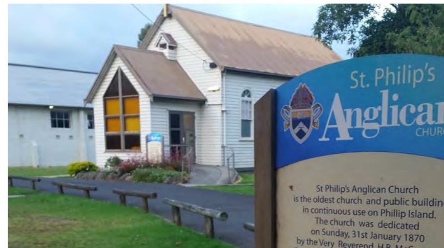
The church does not activate this space
