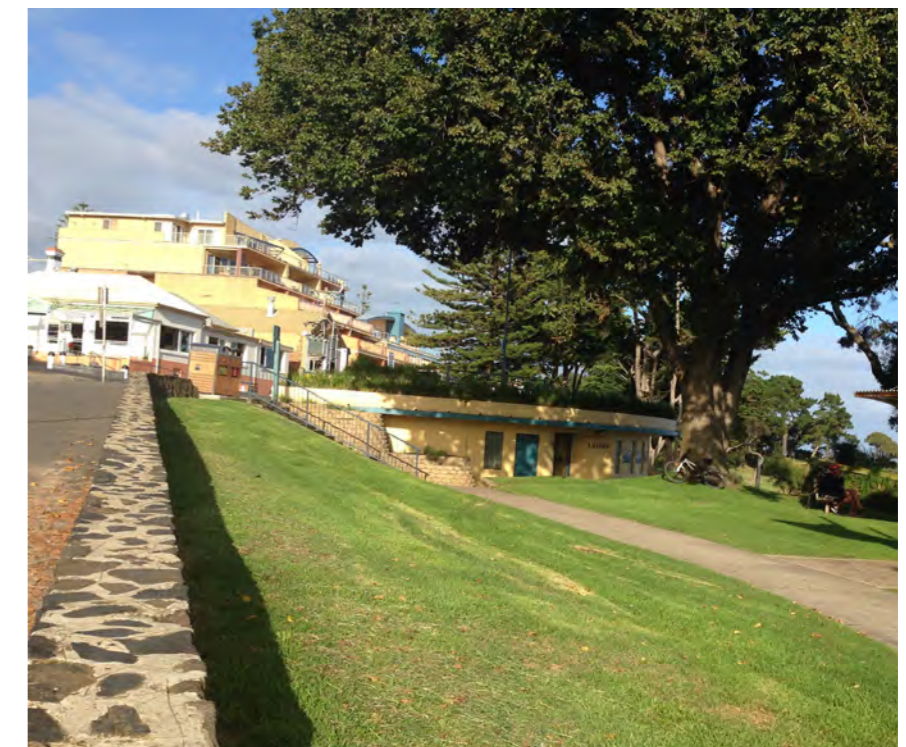
Jetty Triangle areas to be renovated
