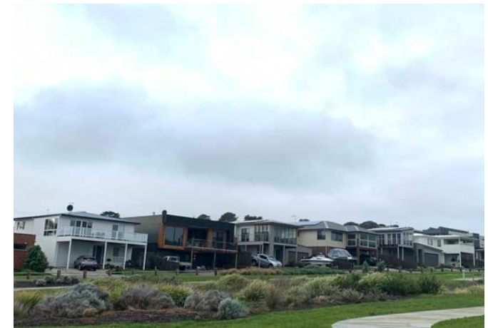
23 New builds with reduced setbacks and building separation - San Remo
