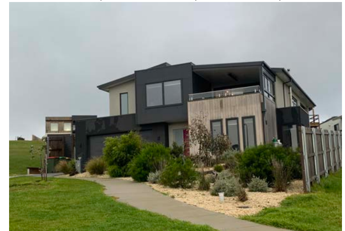
38 Contemporary dwelling featuring varied material finishes -San Remo
