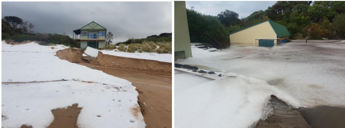
Foreshore area and Wonthaggi Life Saving Club Observation Building, and Council toilet block showing flooding, hail and damage.
