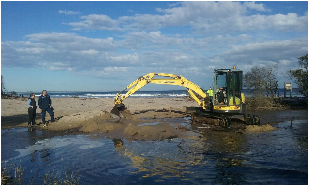
Opening of Wreck Creek, Inverloch to prevent homes flooding
