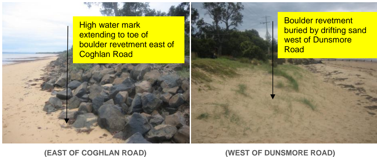
FIGURE 6-4 BOULDER REVETMENTS ALONG STUDY AREA FORESHORE (AUGUST 2010)
