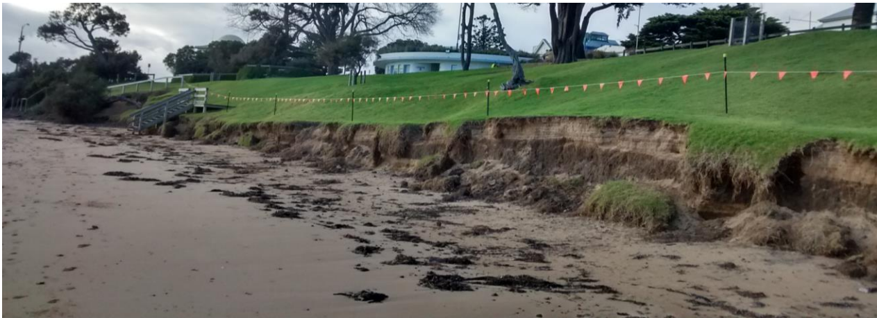
Figure 5-3 Cowes Main Beach Erosion Scarp 3/08/2016 (Bass Coast Shire Council)
