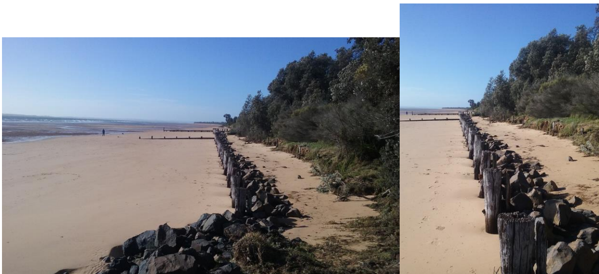
FIGURE 5-10 TIMBER WALL EAST OF ROSE AVENUE 1986 (TOP), 2010 (MIDDLE), 2018 (BOTTOM)
