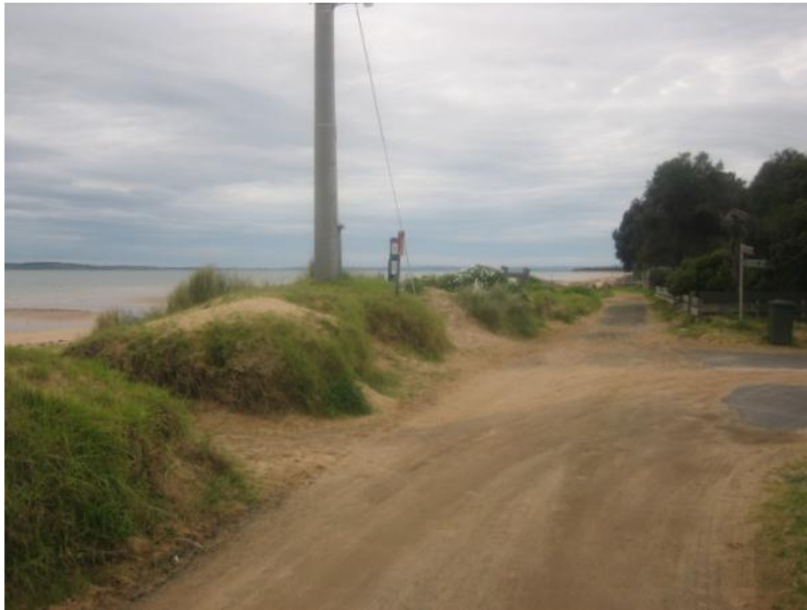
FIGURE 8-4 MULTIPLE BEACH ACCESS PATHS AND WIND-BLOWN SAND IMPACTS NEAR ROSE AVENUE
