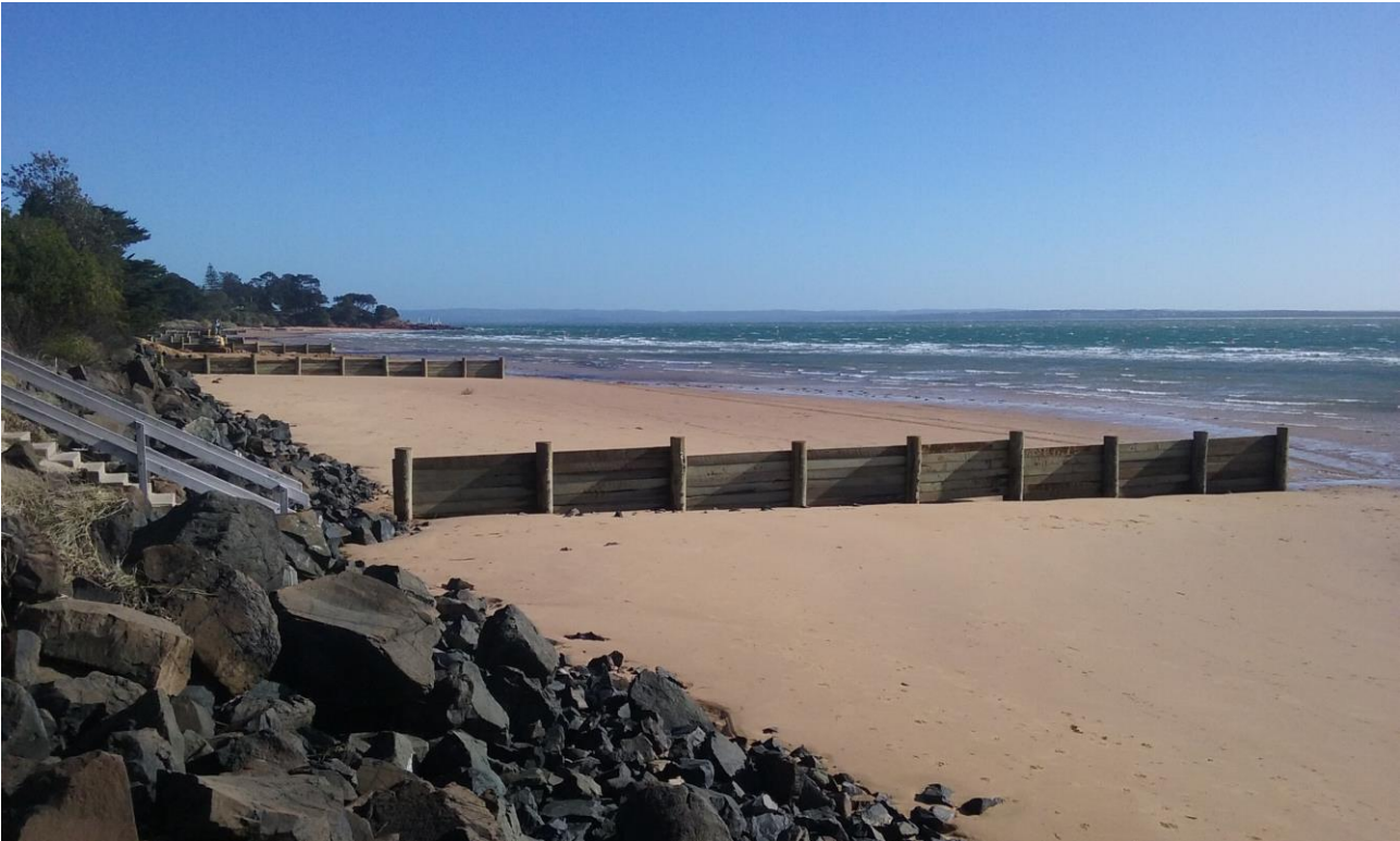
FIGURE 8-1 NEW GROUYNE STRUCTURES INSTALLED NEAR BROUGHTON AVE
