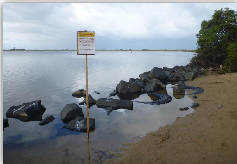
Figure 13 - Rock and tyres used for erosion protection.
