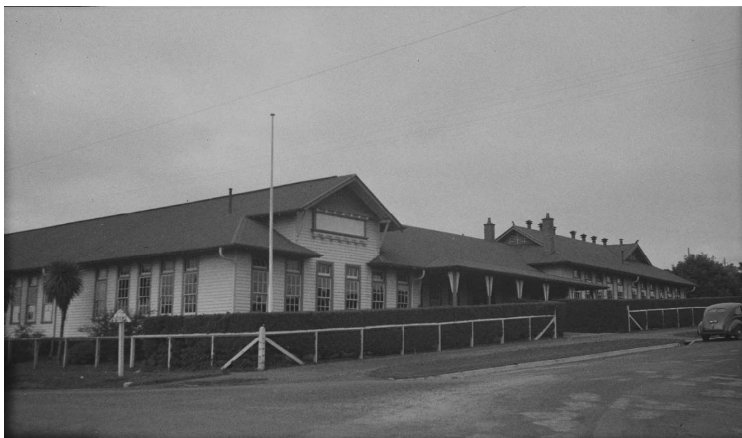
Figure 3.40 Wonthaggi Technical School. (Source: PROV)
