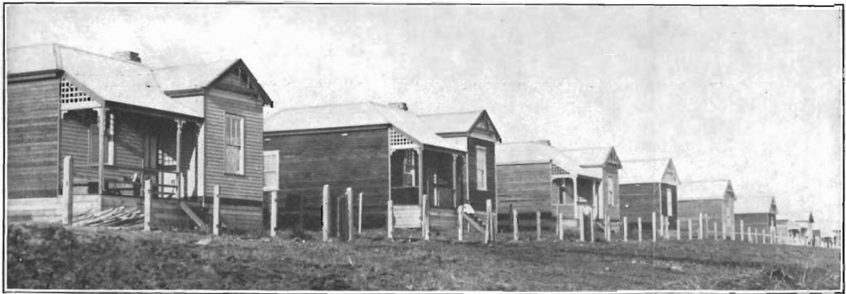
Figure 3.26 A row of miners' cottages in course of construction at Wonthaggi, 1910. (Source: Annual Report of the Manager of State Coal Mines, 1910)
