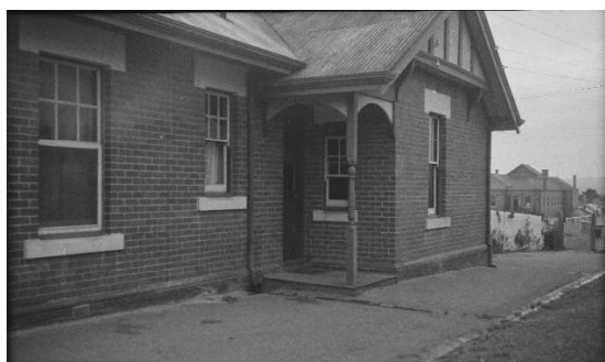
Figure 3.42 Wonthaggi Police Station, erected in 1911. (Source: PROV)
