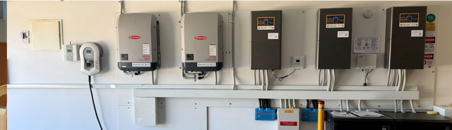
Additional solar PV 25.5 kw and a 2nd EV charging station installed in Werner's home
